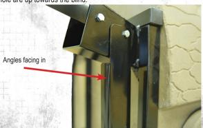
4. Attach the (4) 59 3/4" Center Angle Support in the center of all the legs. Building a "box" frame in the center of the legs. Be sure to have all the angles face the sky when the blind is stood up. All these center angle support brackets attach to the inside of the legs. Once again snug up the bolts but do NOT tighten.
