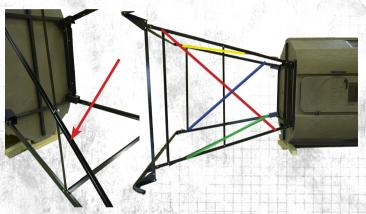
On the bottom sides where your cross braces meet your square tubing braces, dis-attach the square tubing and insert the bolt facing out and attach the cross brace. Then, re-attach the square tubing (Be sure to tighten cross brace before you re-attach square tubing). Snug up each bolt but do not tighten completely.
